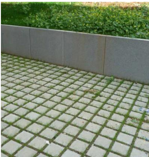
Pavés béton joints gazon
